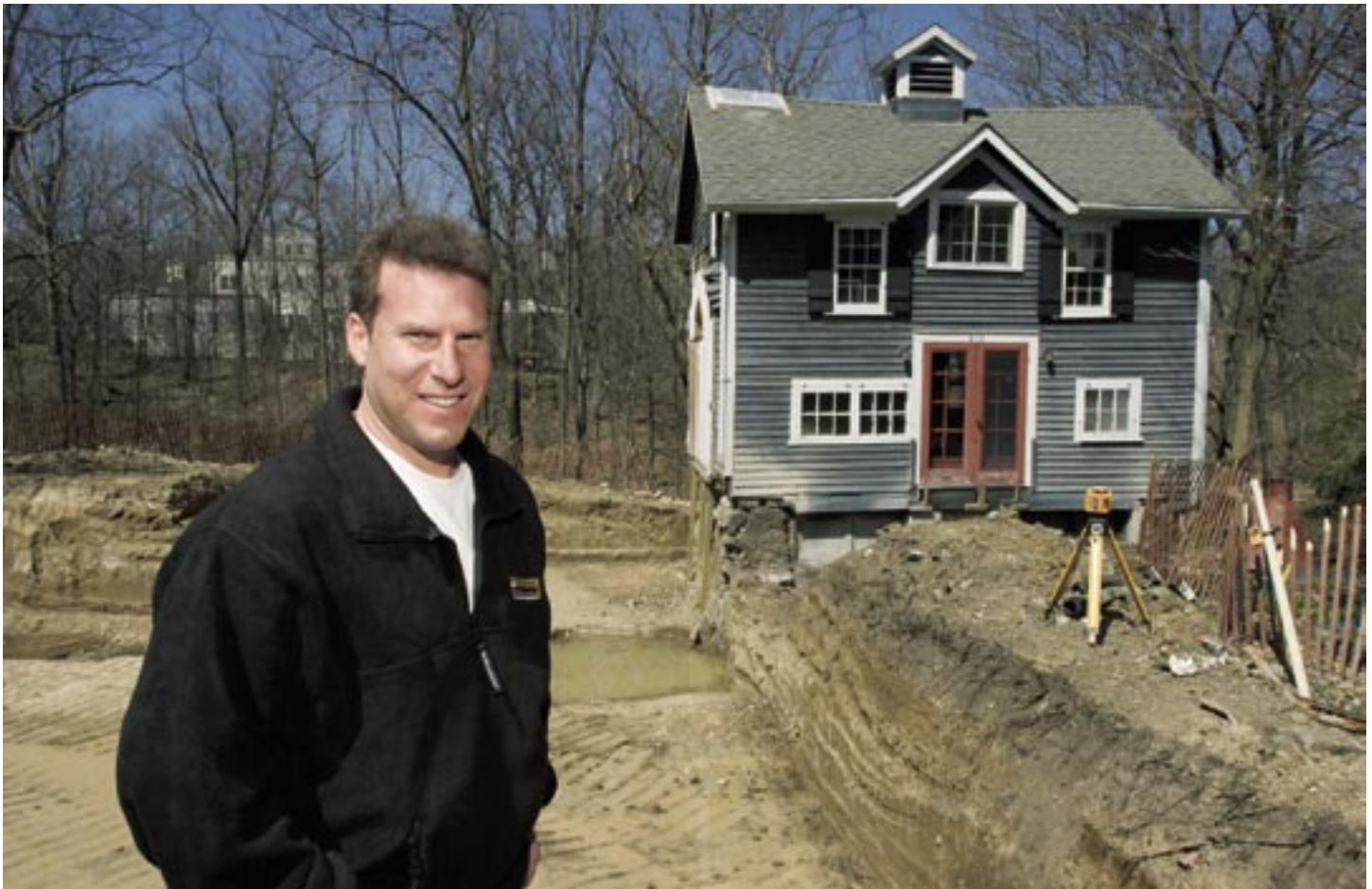
On location of a circa 1880 stable which Z Construction will be restoring and adding on to.
